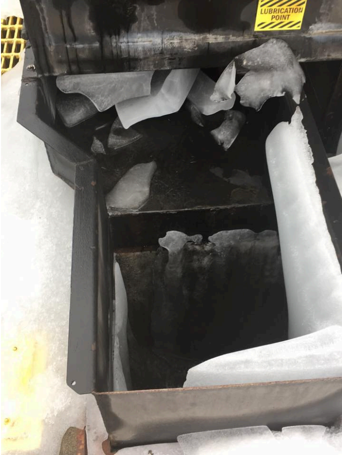
Photo 5: Debris Trough Exit Again.
